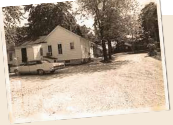
The original restaurant in Glenwood circa 1970
